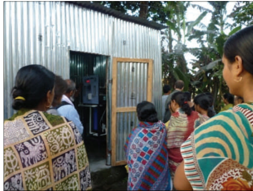
Visit of the water purification unit, Randhamali, West-Bengal, March 10th, 2012.
